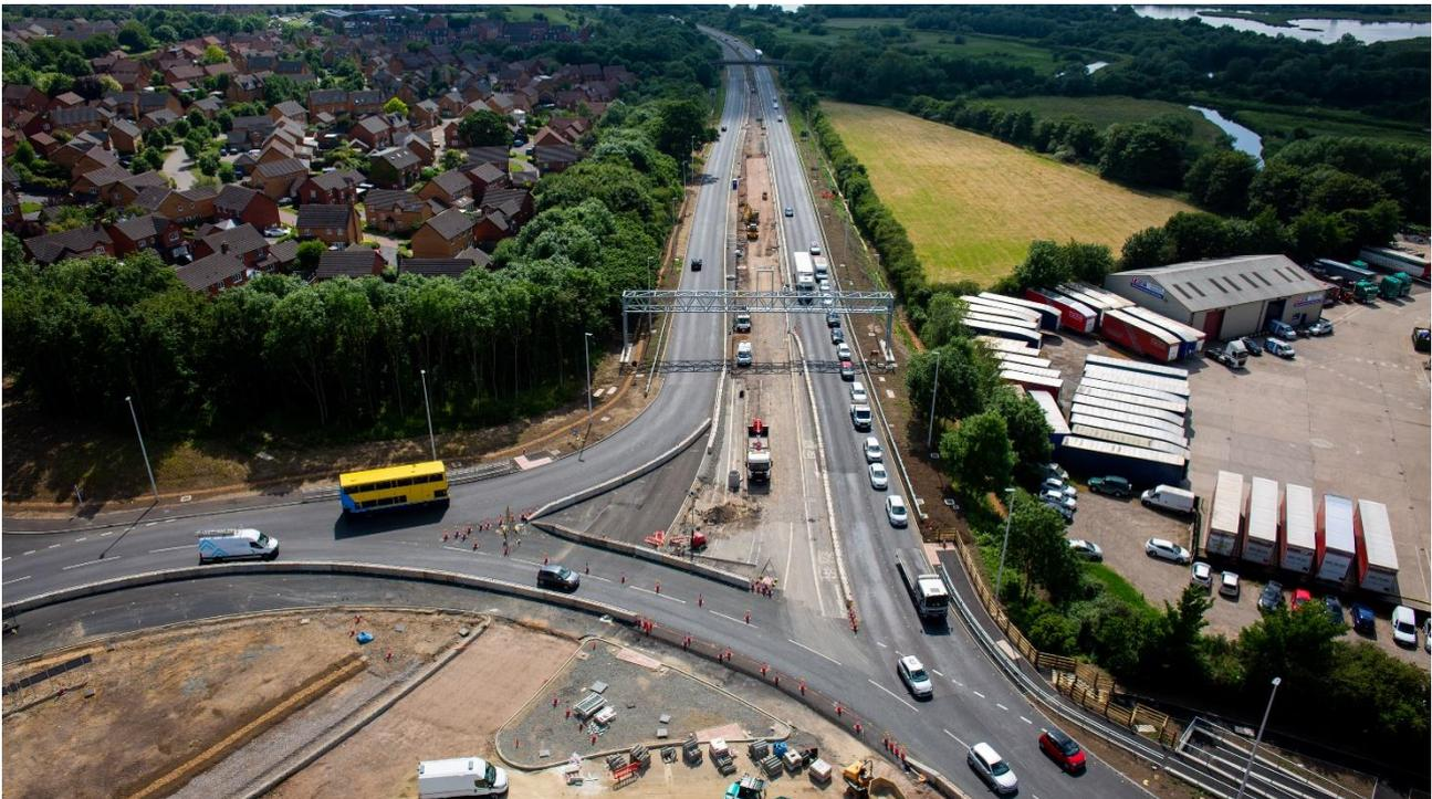
*Image shows gantry installation on the A45 Western arm*
