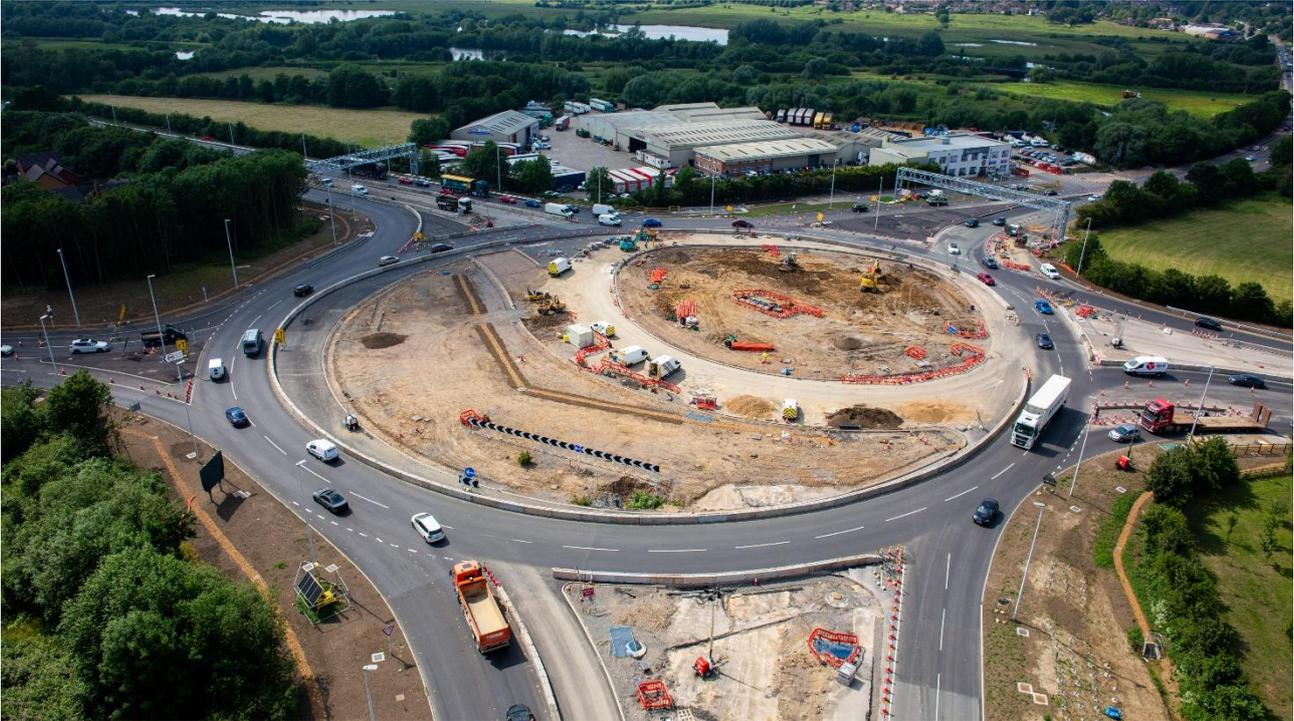
*Image shows the outline of the new half hamburger roundabout design – the A45 traffic will flow through the middle section of the roundabout - June 2021*
