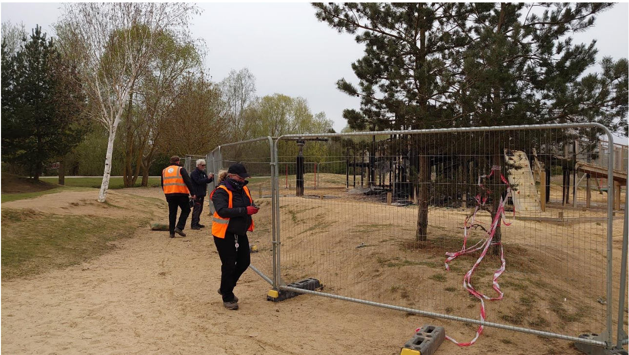
Image shows the security fencing being installed at Stanwick Lakes
