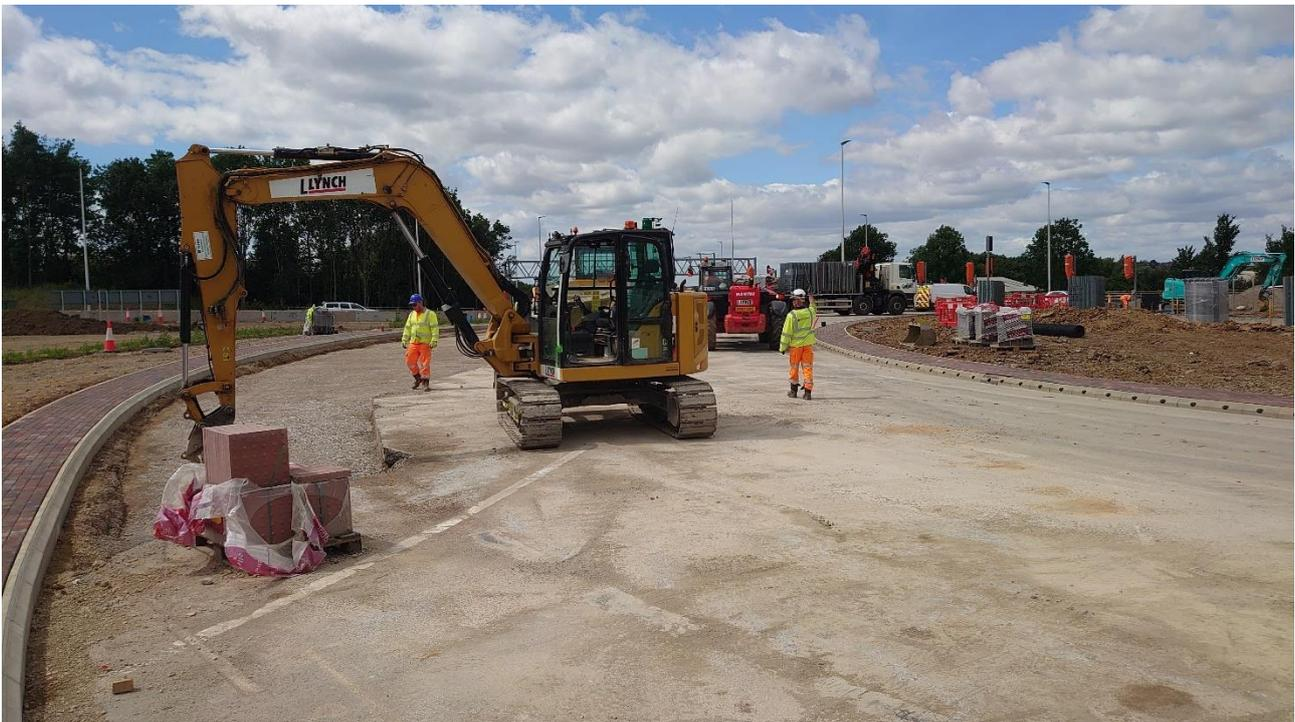
*Image shows the kerbing and new block paving line that defines the new A45 carriageway space between the half hamburger and central island.*
